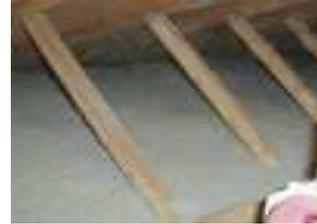
Shortly after installation much of the moisture added for installation will evaporate. The insulation will “shrink” a small predetermined amount and will stabilize to the proper depth to yield the specified R-value.
